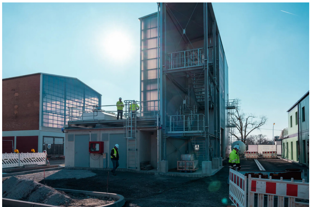
Caphenia's pilot plant in Frankfurt, Germany began construction in 2024. 12
